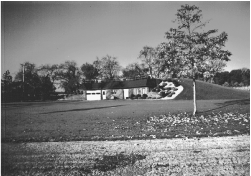
Figure 13.7 Earth shelter on a flat site with berm. (Davis Caves Construction, Inc.)
